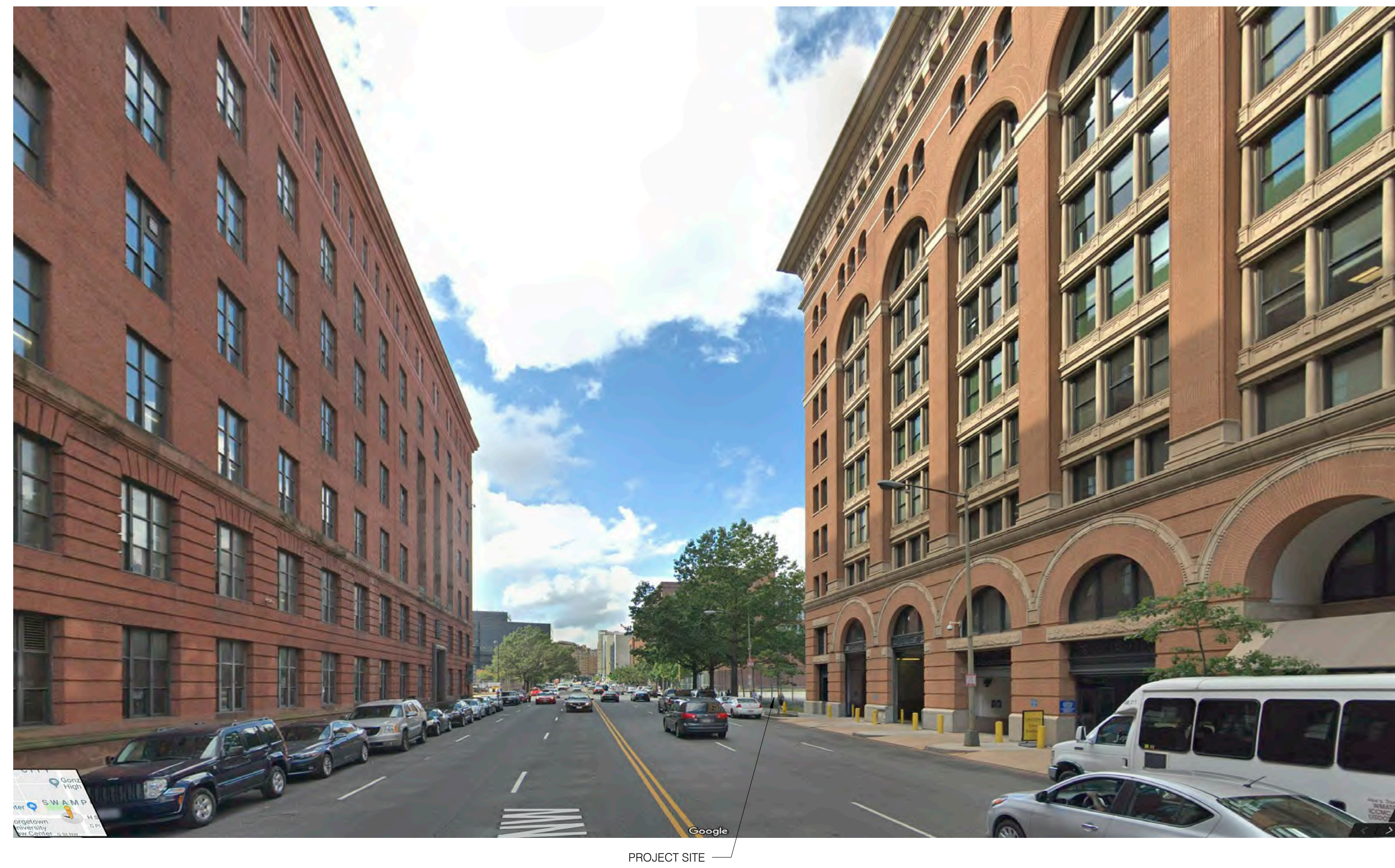
2 SITE PHOTO - H STREET LOOKING WEST
